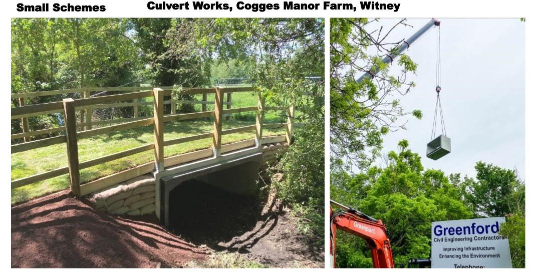
This project involved the clearing of an overgrown culvert at a historically protected farm in Witney. Greenford created and installed a strong culvert structure to allow water to continue to flow effortlessly under the bridge.
