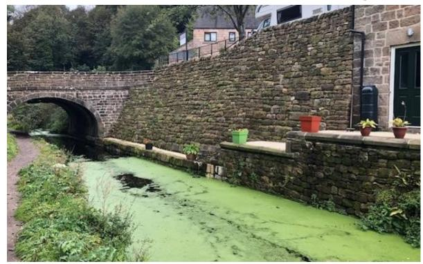
Greenford carried out the work on this historical flood gate system built in the canal walls and bed. The remains were discovered during the initial excavation which Greenford rebuilt and replicated in order to form the new wall.
